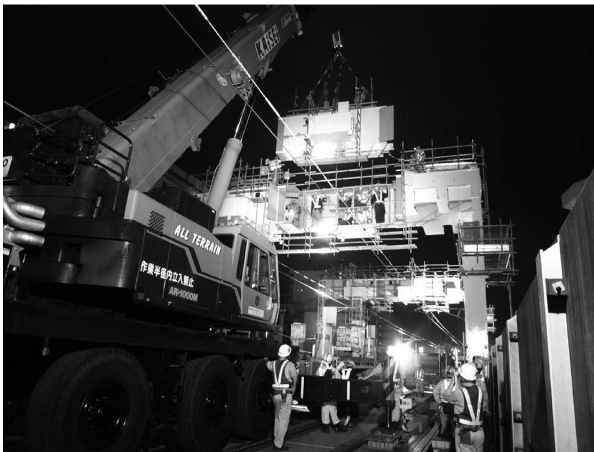
100-tonne all-terrain crane erecting steel frame
