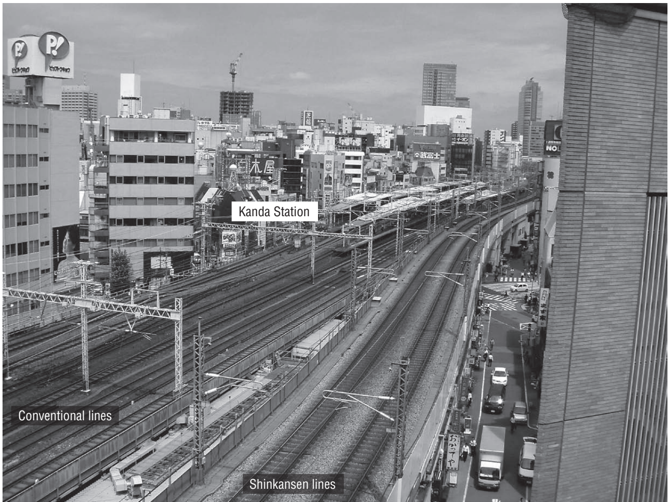
Conventional lines and Shinkansen line located adjacently.
