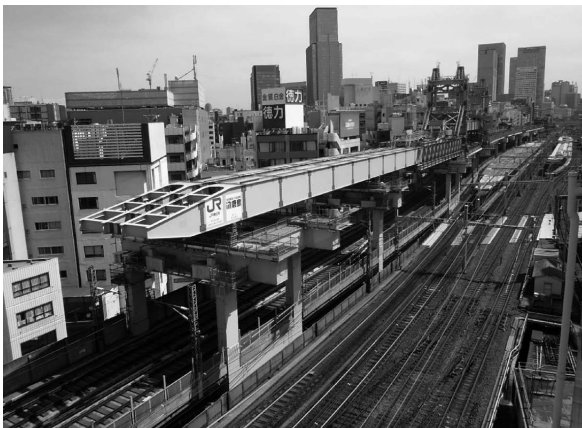
Girder erection in progress
