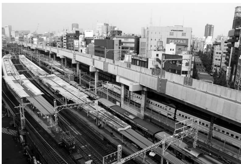
Construction of Ueno–Tokyo Line near Kanda Station
