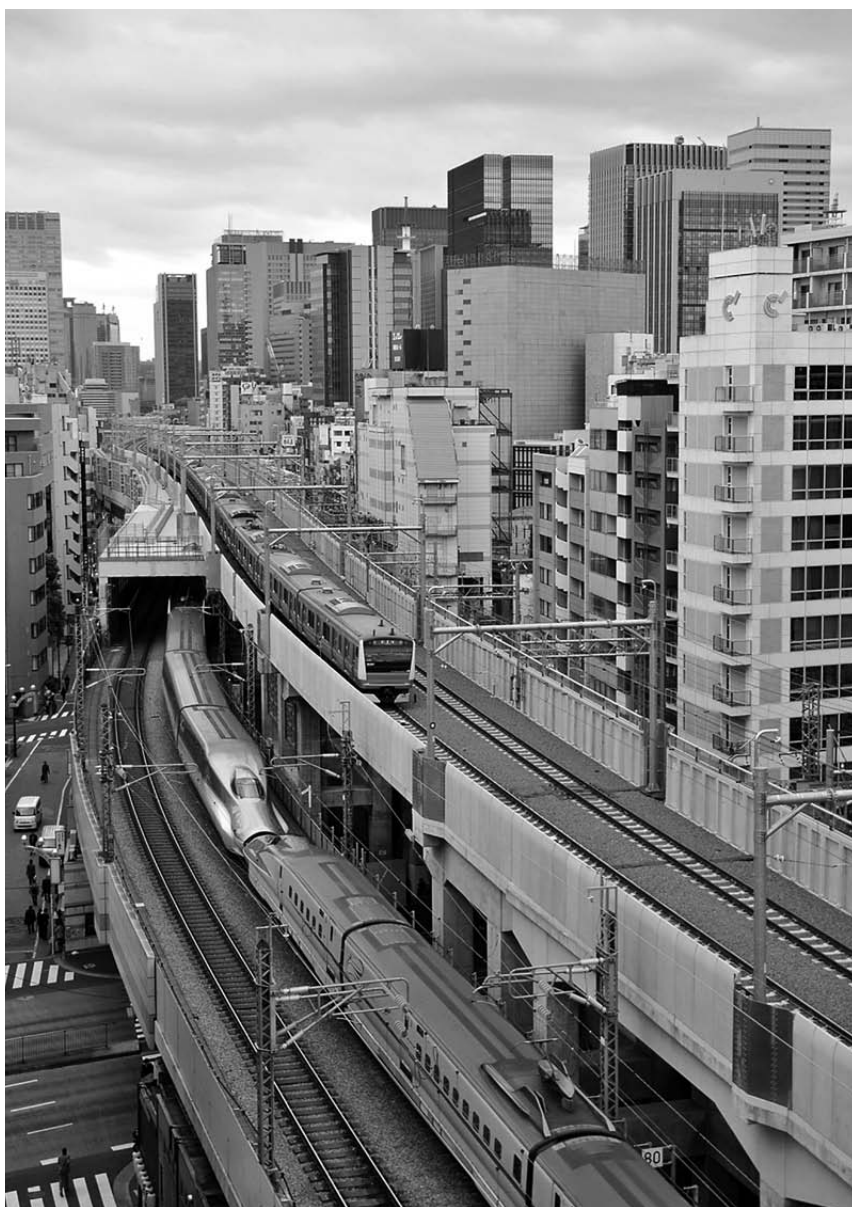
Completed Ueno–Tokyo Line running near Kanda Station
