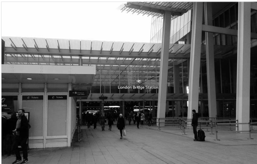
London Bridge Station was improved for Thameslink opening
