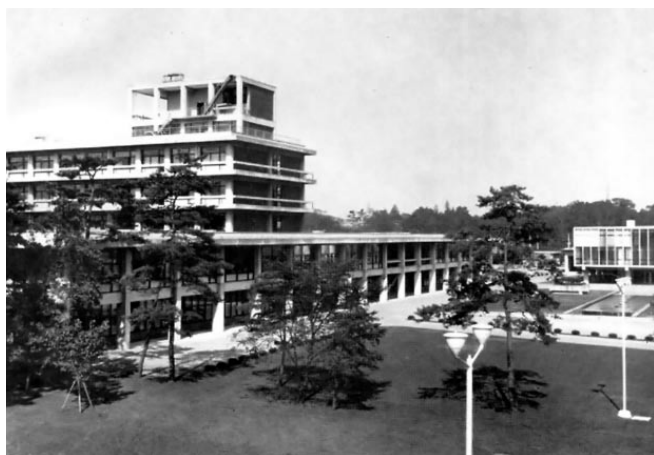
New RTRI building Completed in 1959
