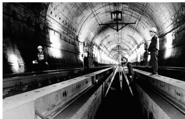
Surveying in Seikan Tunnel
