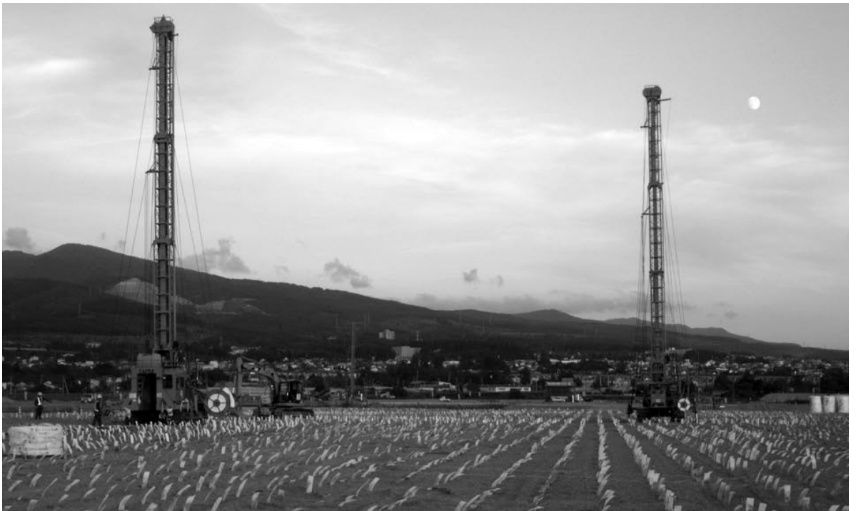
Hakodate General Rolling Stock Yard Embankment (Vertical Drain)
