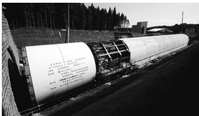
Tsugaru-Yomogita Tunnel Shield Borer
