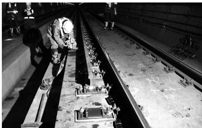
Three-Rail Track Laying
