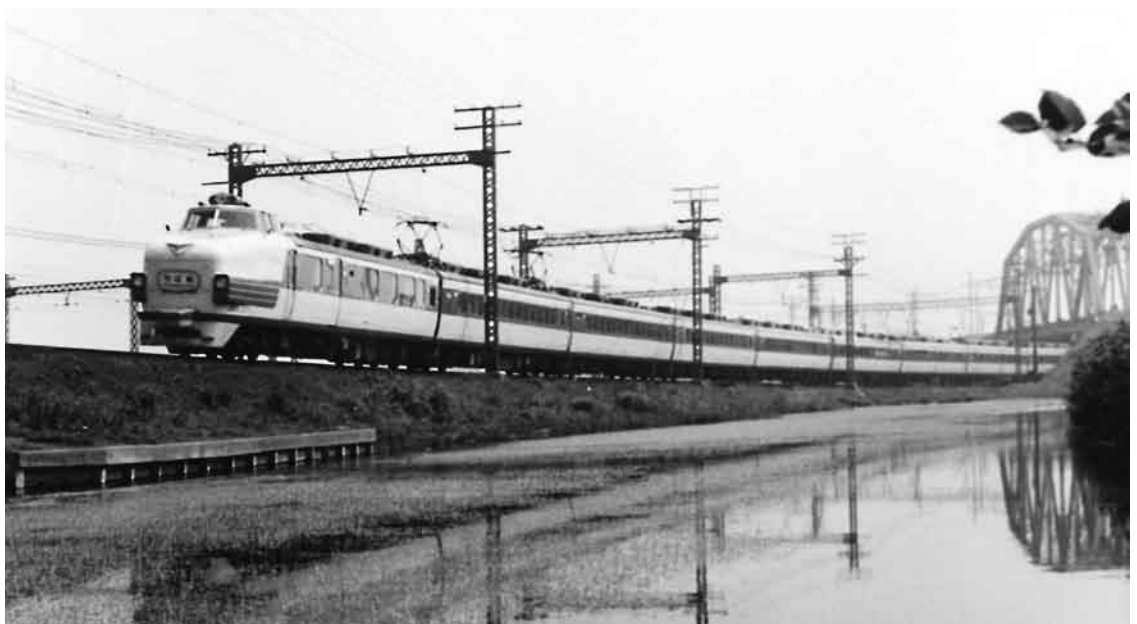
The Series 151 DC EMU running 556 km between Tokyo and Osaka in 6.5 hours from 1958 was the culmination of new technologies developed by private railways and manufacturers from around 1950 (The Railway Museum)
