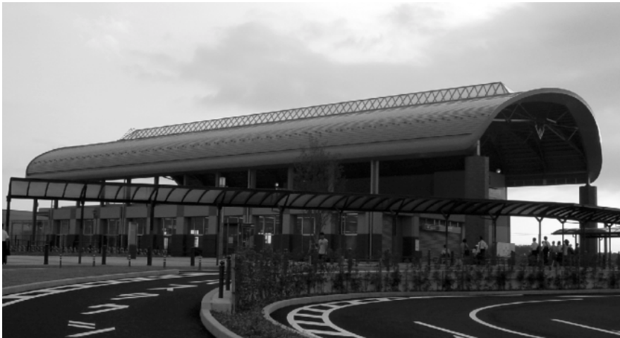
Miraidaira Station external view
