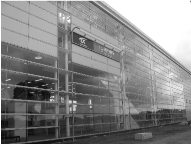
Exterior wall of hybrid structure
