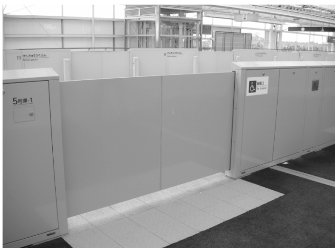
Platform screen with moveable gate
