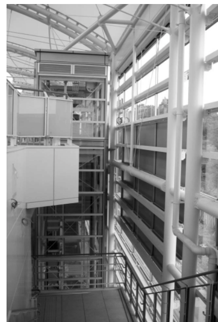
Staircase in hybrid structure (constructed adjacent to building façade) (JRTT)
