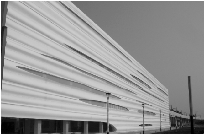
Kashiwanoha Campus Station façade
