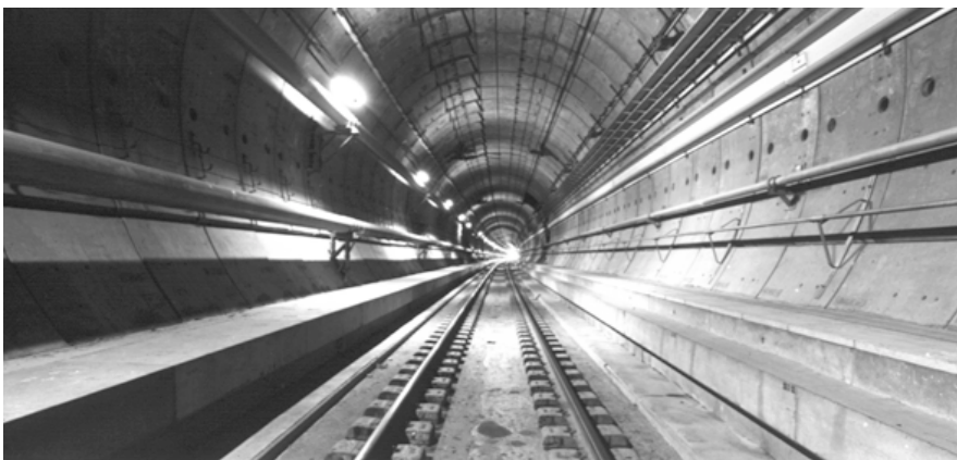
One of running tunnels
