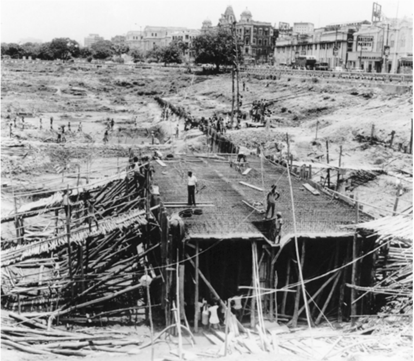
Calcutta Subway under construction by cut-and-cover method (top). Completed subway station and domestically built trainset (opposite page left). Busy platforms (opposite page right and bottom left) and crowded train (bottom right) of Calcutta Subway. (Photos: Author)
