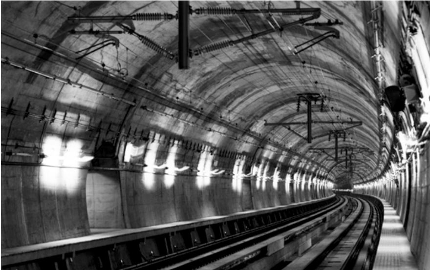
Seikan Undersea Tunnel
