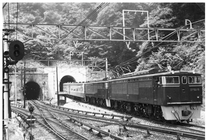
EF63 Electric loco used exclusively on steep grade at Usui Pass
