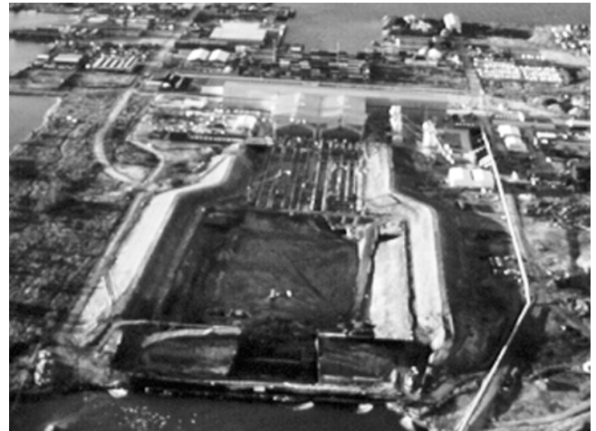
Tunnel element factory under construction with large floating basin in foreground (Øresundskonsortiet)
