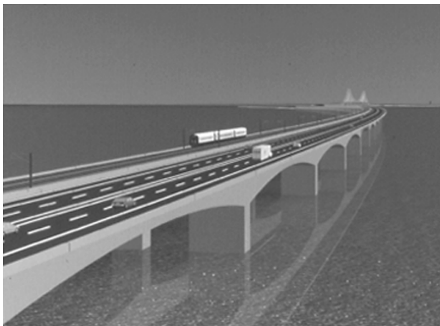
The West Bridge is a low motorway and railway concrete bridge.
