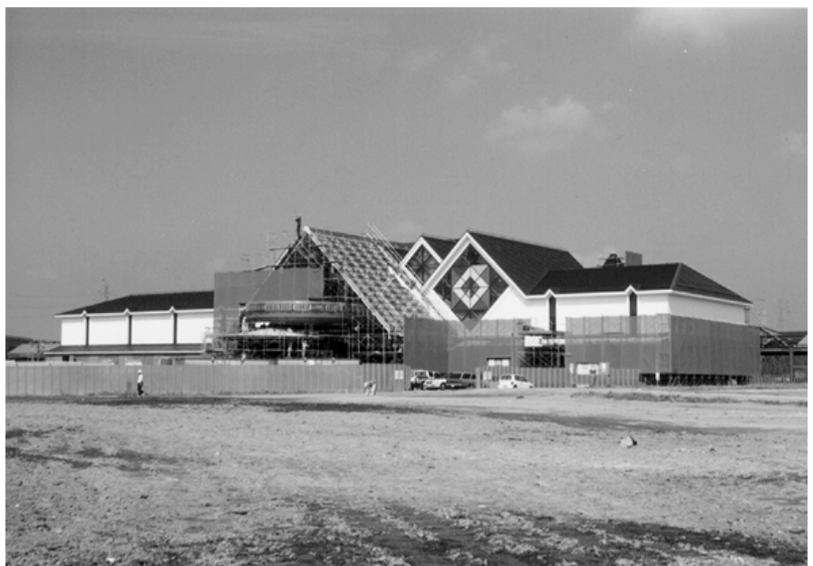
Saku Station under construction on Hokuriku Shinkansen
