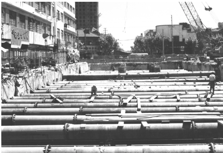
Cut and Cover Construction of Shanghai No. 1 Subway Line
