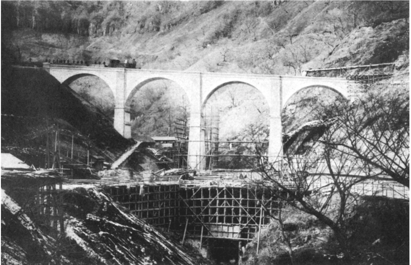
■ The Usui Viaduct under construction at a 1:15 grade between Yokokawa and Karuizawa. The track used a rack-and-pinion system. The viaduct is now preserved as a historic monument and has been replaced by an alternative route. Reprinted from RAILWAYS AND ROLLING STOCK IN JAPAN
