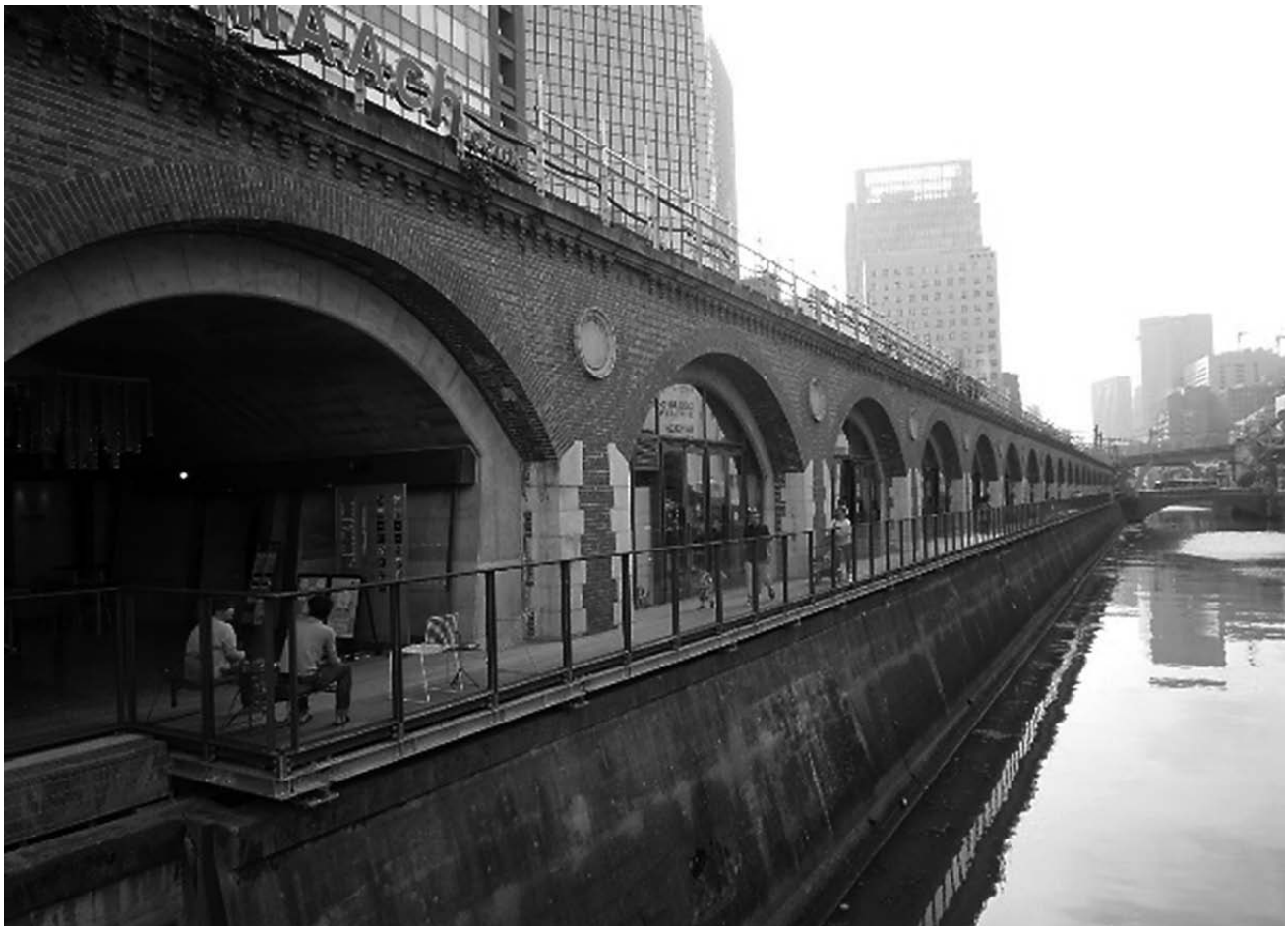
Under-viaduct space commercial facility near Ochanomizu Station on Chuo Line (The space under an old brick arch viaduct was renovated with a through passage in shops and along the river) (Author)
