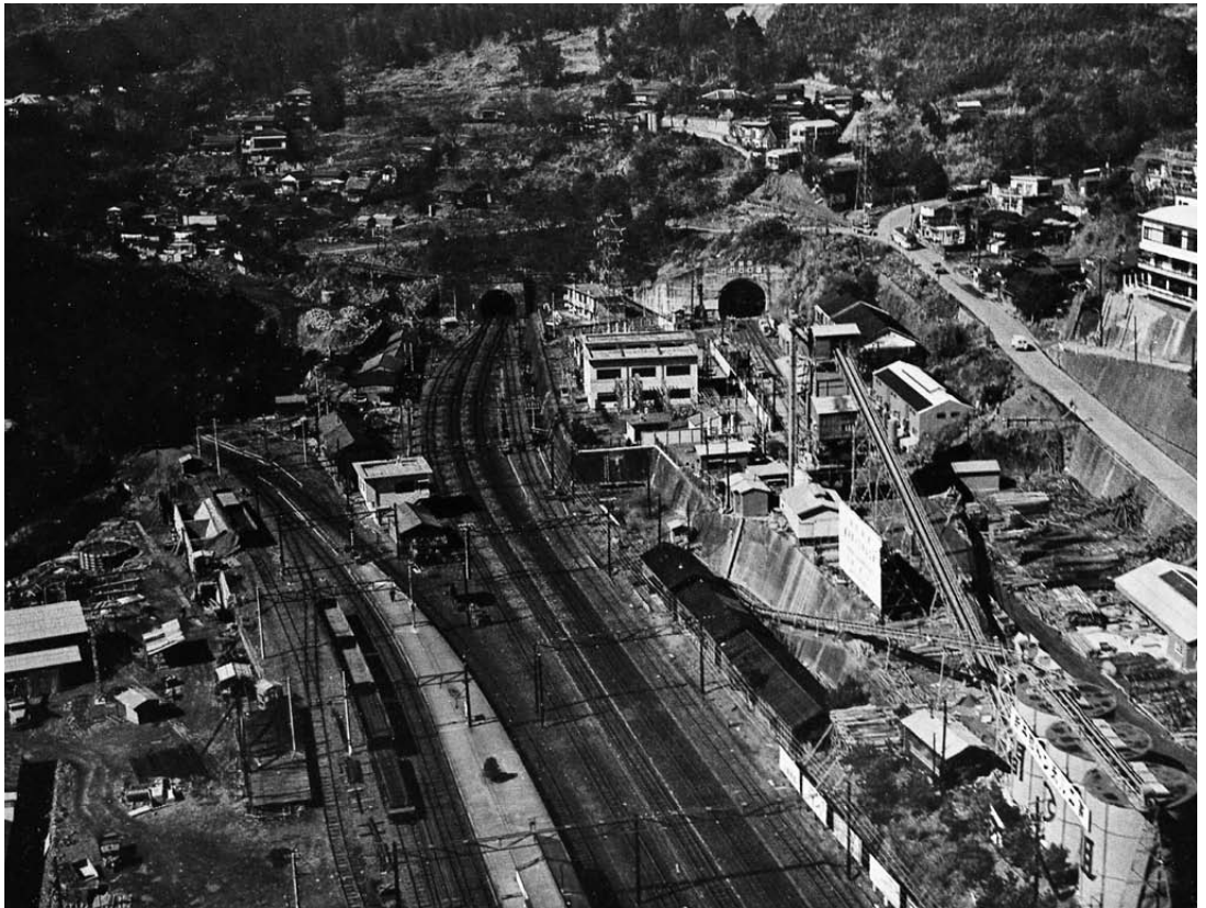
Tokaido Shinkansen Shin-Tanna Tunnel (1964) (parallel to conventional-line Tanna Tunnel on north side)
