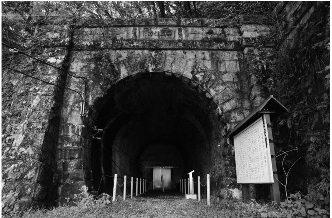
Osakayama Tunnel built solely by Japanese engineers (1880) (now preserved as railway memorial)
