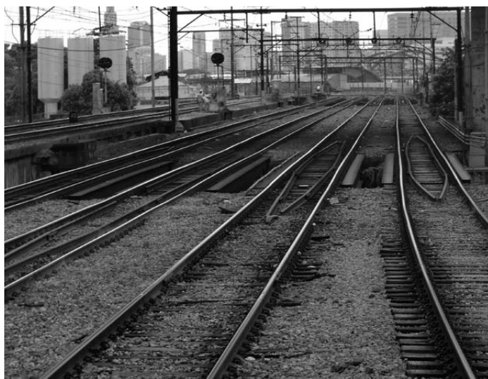
Track gauge widening (left) and dilapidated carriages (right)
