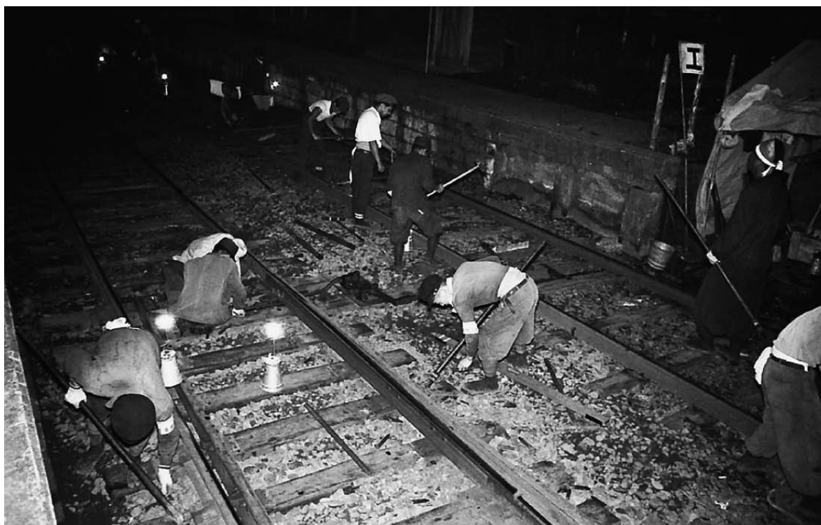
Construction to change gauge of Keisei Electric Railway
