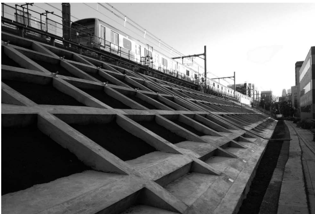
Large earthquake countermeasures (aseismic reinforcement of embankments)
