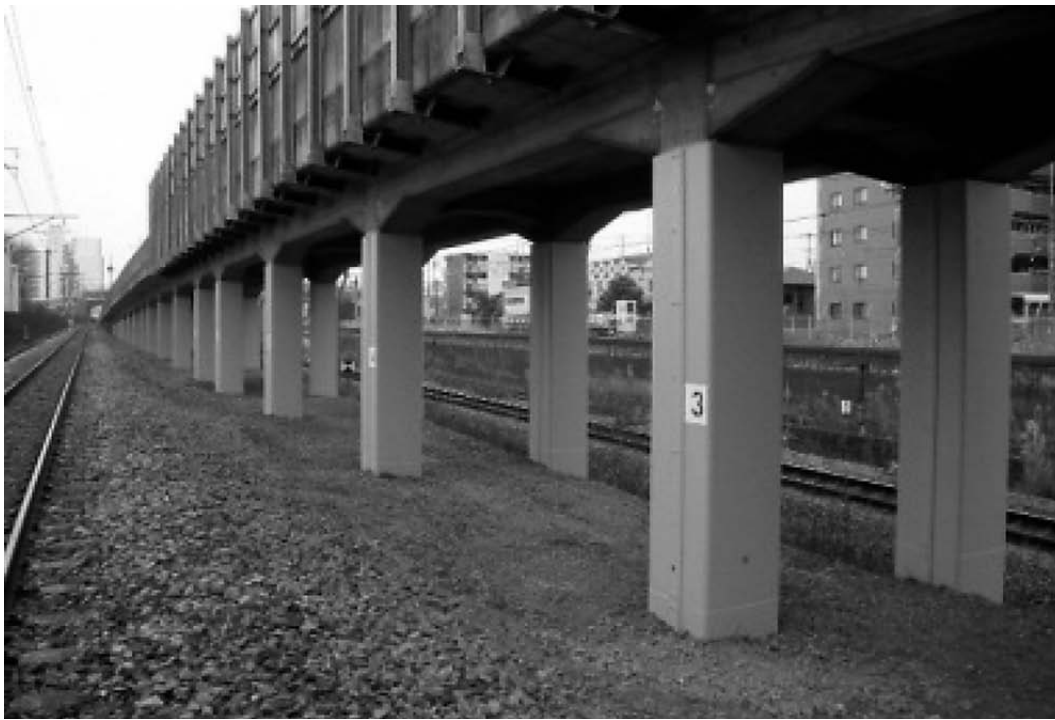
Large earthquake countermeasures (aseismic reinforcement of viaducts)
