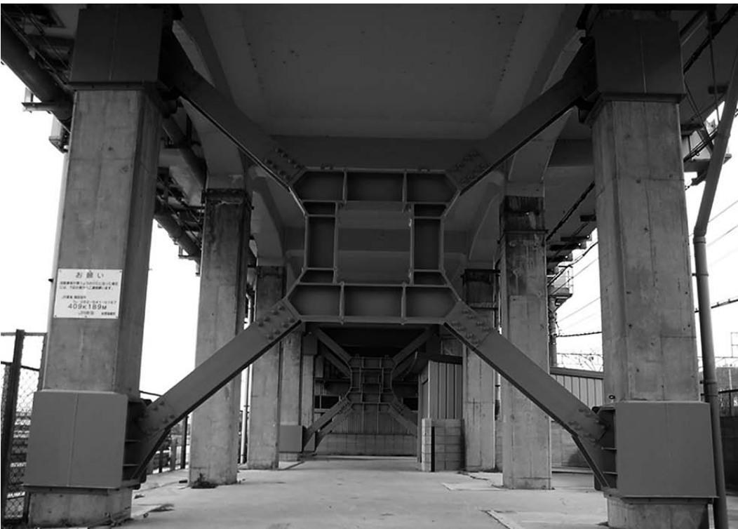
Countermeasures against viaduct displacement
