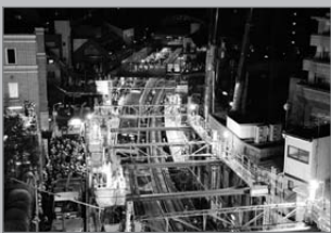
Construction to switch to underground track near Daikanyama Station (Tokyu Corporation)
