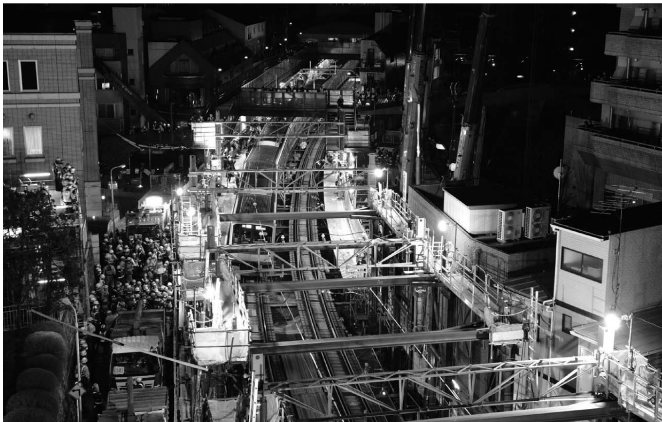
Construction to switch to underground track near Daikanyama Station
