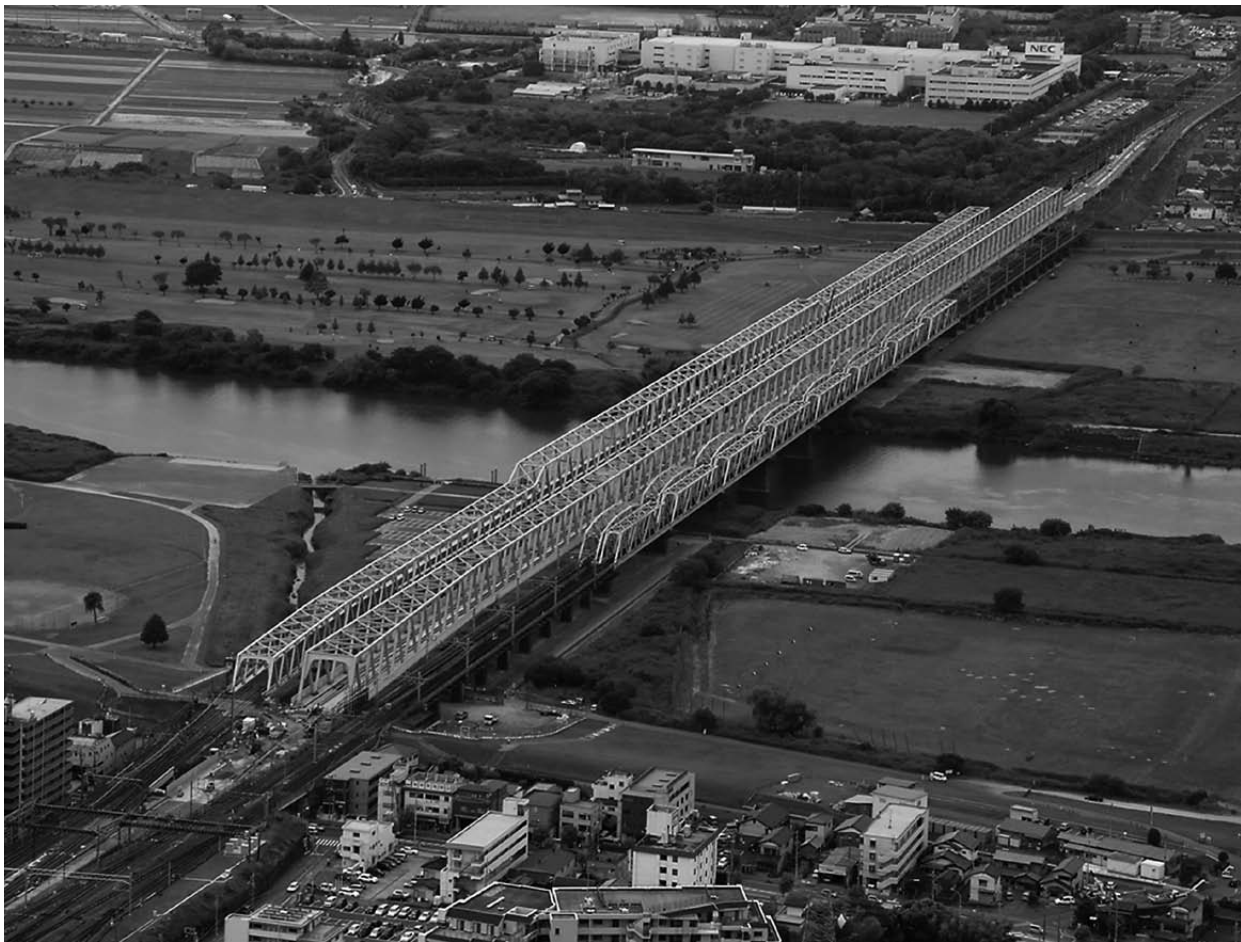
Replacement of Tone River Bridge
