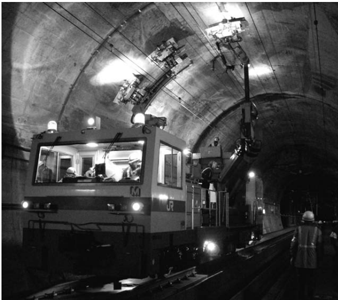
Concrete Lining Inspection Car (CLIC)
