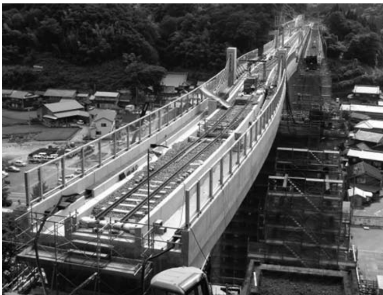
Lateral motion of girders and turning erection method (before)
