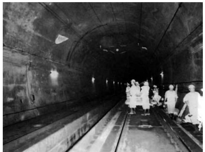
Concrete falls from Fukuoka Tunnel lining of San'yō Shinkansen in 1999 (JR West)
