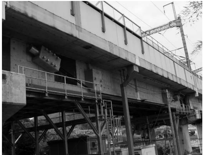
PC External cable tension monitoring system
