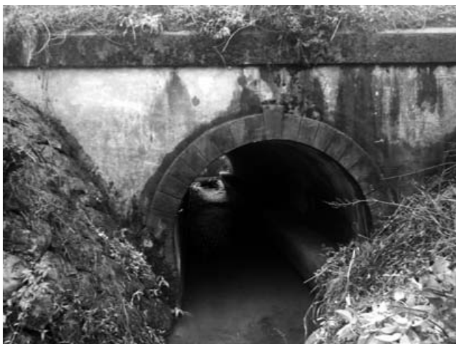
Shimadagawa Bridge, first RC railway bridge in Japan (JR West)
