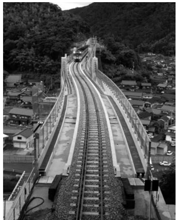
Lateral motion of girders and turning erection method (after)
