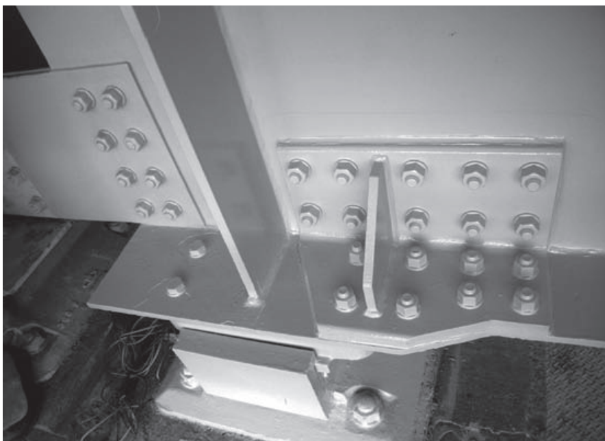
Reinforcement by patch plates
