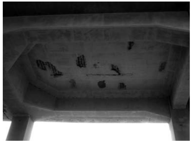
Hammered-off areas under viaduct slab
