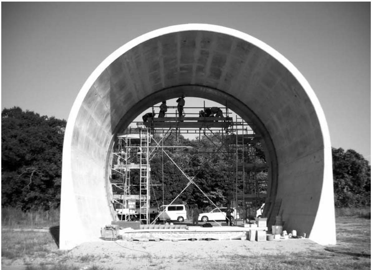
Full-scale tunnel for developing additional inner lining
