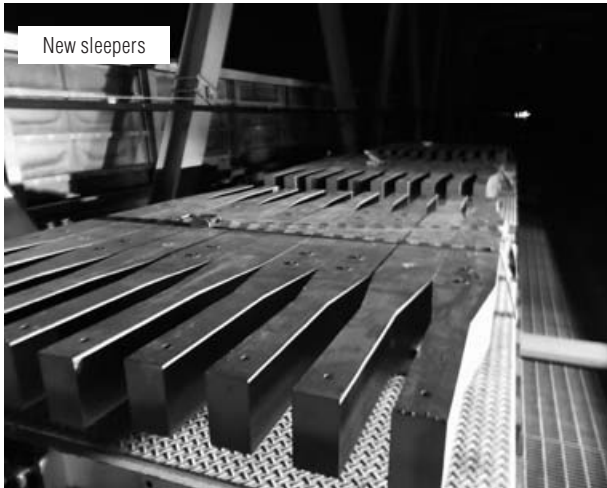
Figure 11 Inserting Sleepers
