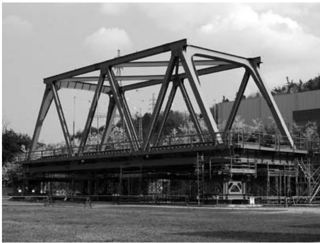
Full-scale truss model (Komaki Research Centre)
