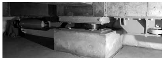
Seismic rubber isolators and oil dampers (JR East)
