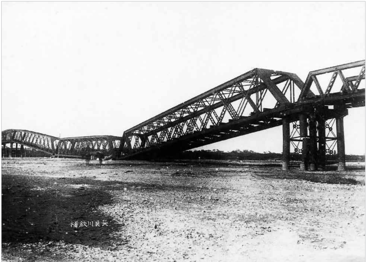
Railway Damage due to Nobi Earthquake (Nagaragawa Bridge) (1891)
