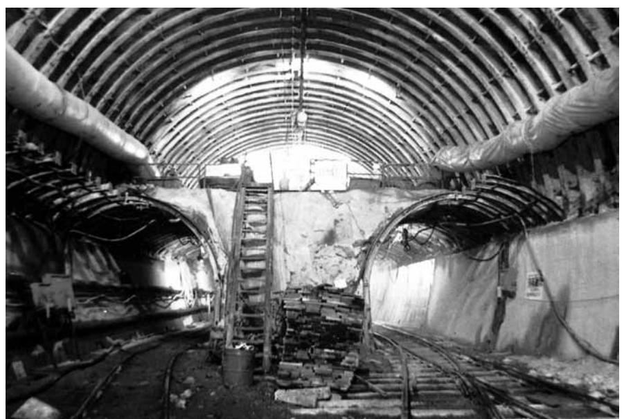
Seikan Undersea Tunnel Construction (1983)
