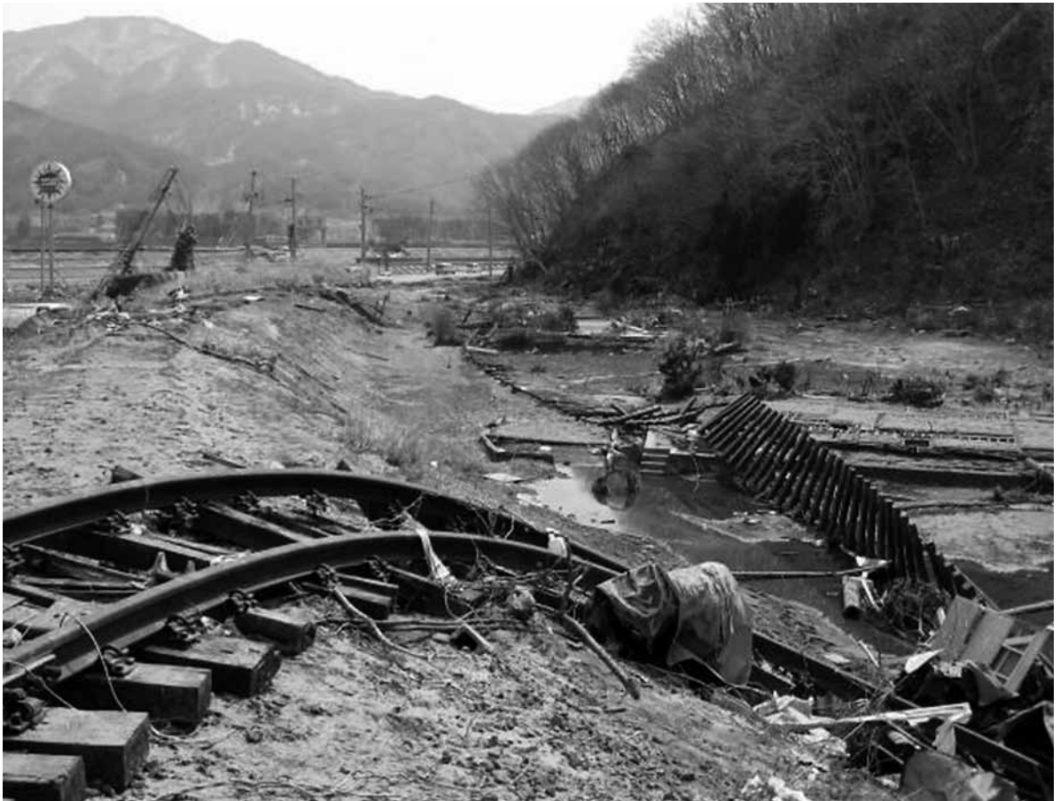
Railway Damage due to Great East Japan Earthquake (2011)
