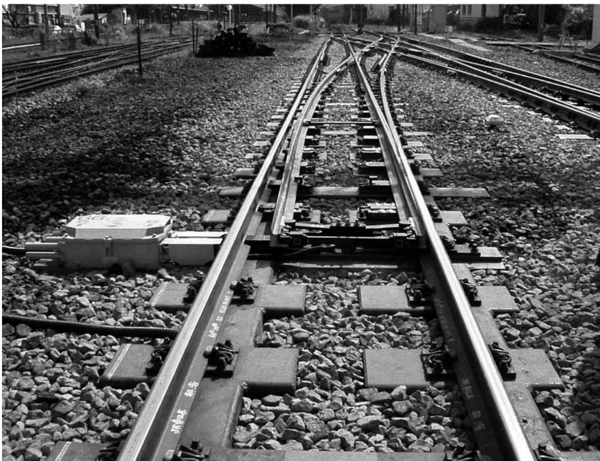
Next-generation turnout and grid type sleepers (JR East)
