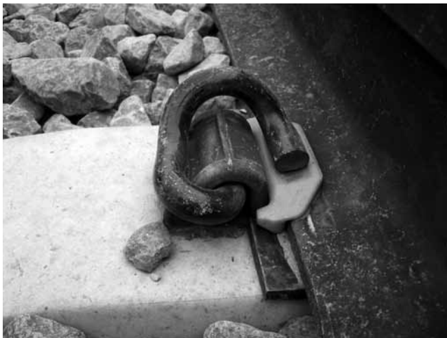
Spring clip type rail fastening system developed in UK (JR East)
