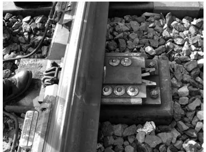
Ball bearing base plate developed in Sweden (JR East)
