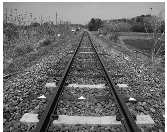
Low-cost PC sleepers for local lines
