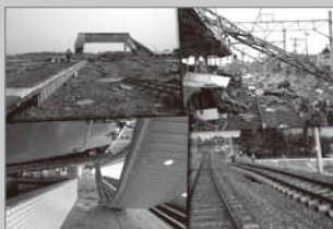
Clockwise from bottom left: earthquake damage at Sendai Station, and tsunami damage at Shinchi Station (top left), Nobiru Station (top right), and sections between Mito and Katsuta. All of the above photographs are courtesy of JR East.
