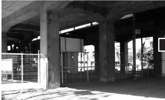
Aseismic reinforcement of viaducts
