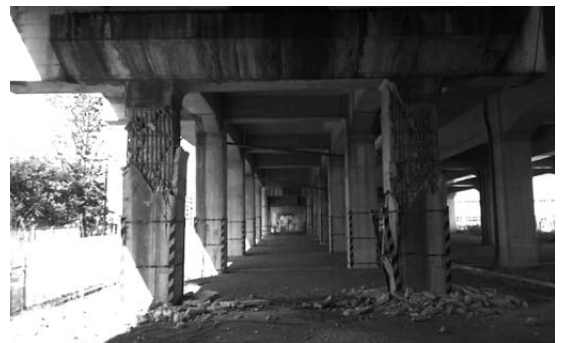
Damage to viaducts
