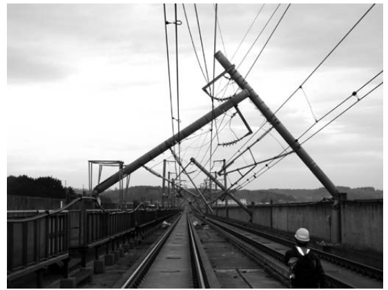
Damage to electric poles
