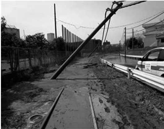
Liquefaction on Echujima Line (JR East)
