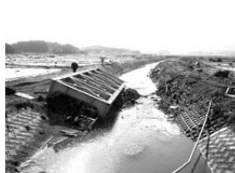
K [Bridge girders swept away] Joban Line between Shinchi and Sakamoto
