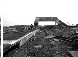
L [Track swept away] Joban Line in yard at Shinchi
