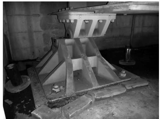
Damage to supports
