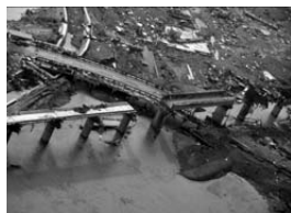
H [Bridge girders swept away] Kesennuma Line between Rikuzen-Koizumi and Motoyoshi
