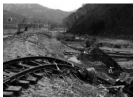
C [Track swept away] Yamada Line between Sokei and Tsugaruishi
