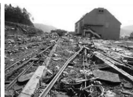
I [Track swept away] Ishinomaki Line in yard at Onagawa
