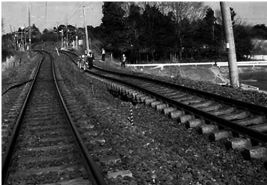
Embankment subsidence between Mito and Katsuta on Joban Line (JR East)
