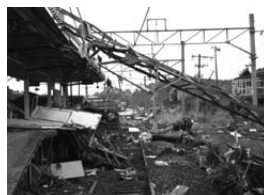
J [Roadbed swept away] Senseki Line in yard at Nobiru
