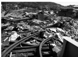
E [Track swept away] Ofunato Line in yard at Hosoura
