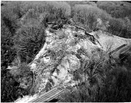
Landslide between Toyohara and Shirasaka on Tohoku main line (JR East)
