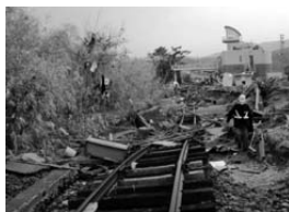
G [Track swept away] Kesennuma Line in yard at Oyakaigan
