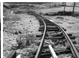
B [Track swept away] Hachinohe Line between Shukunohe and Rikuchu-Yagi
