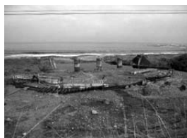
A [Bridge girders swept away] Hachinohe Line between Shukunohe and Rikuchu-Yagi
