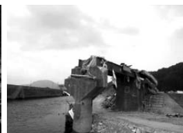
D [Bridge girders swept away] Yamada Line between Rikuchu-Yamada and Oriokasa
