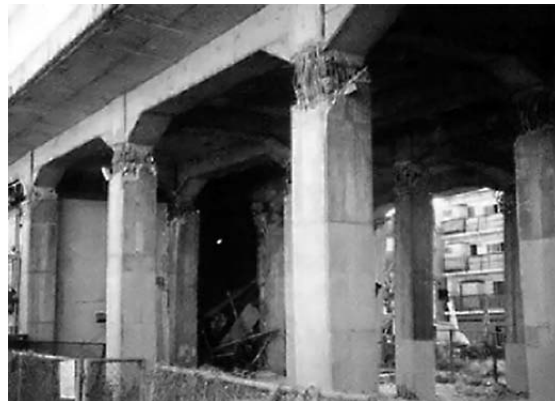
Flexural failure
