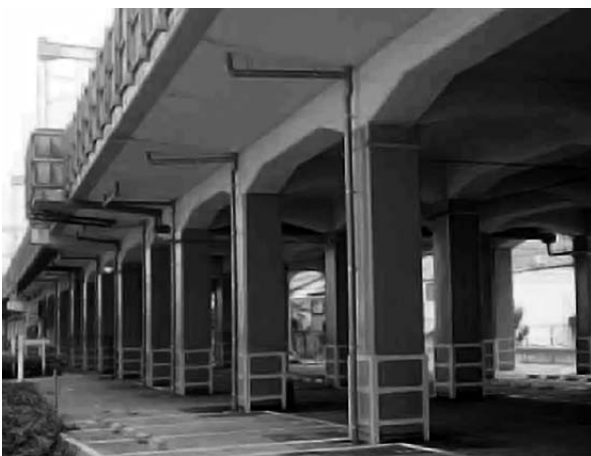
Figure 5 Standard Reinforcing Method for Viaducts
