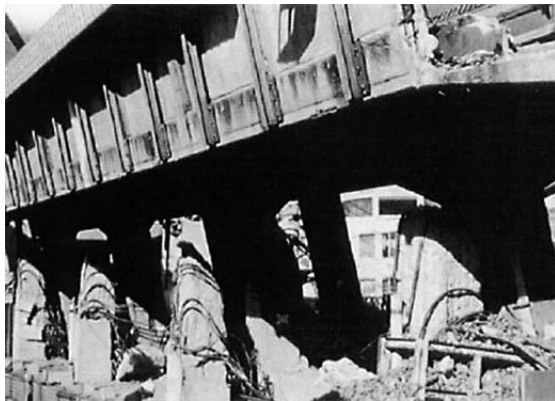
Shear failure
