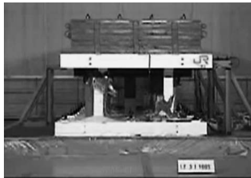
Non-reinforced (after shaking)
