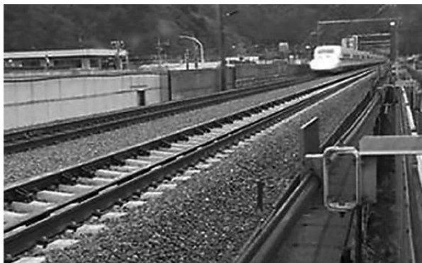
Figure 17 Derailment Prevention Guards on Main-Line Track
