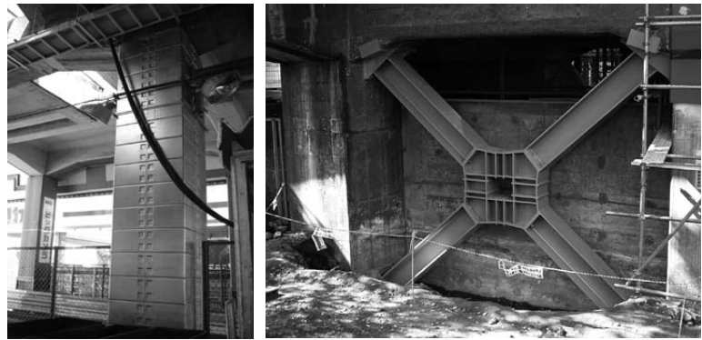
Assembly of steel plates
