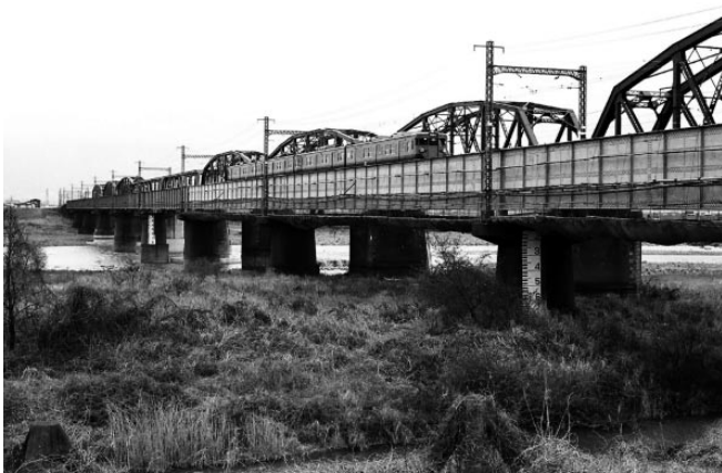
Three-span continuous half through plate girder of up line of Fujigawa Bridge (Author)
