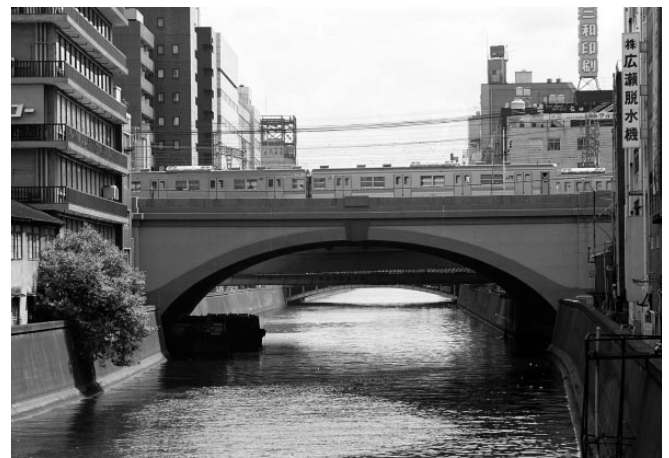
Kandagawa Arch Bridge (Tohoku Line, Tokyo)
