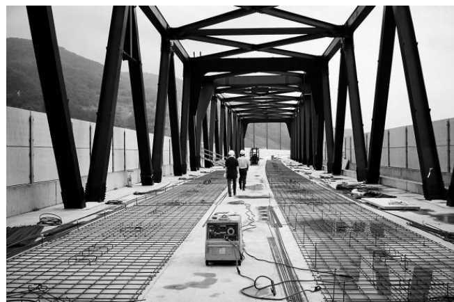
Saigawa Bridge on Hokuriku Shinkansen during bridge decking construction (Author)
