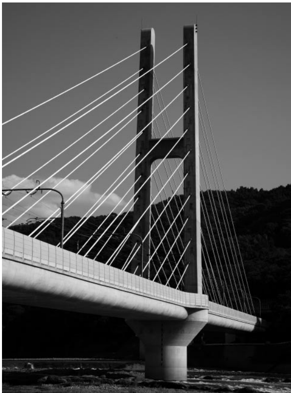
No. 2 Chikumagawa Bridge
