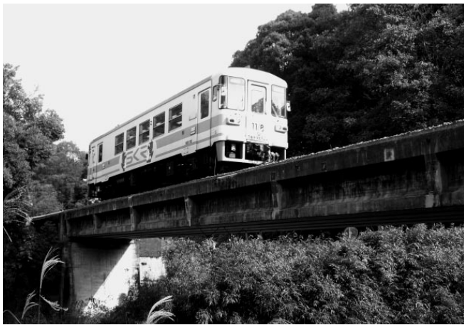
Daidogawa Bridge—start of PC bridge advancement (Shigaraki Kougen Railway)
