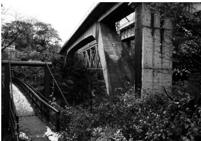
No. 8 Tonegawa Bridge down line (Author)
