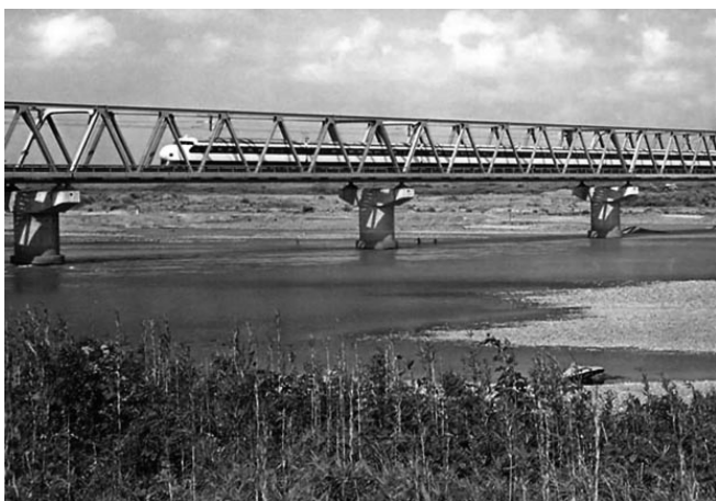
Tokaido Shinkansen truss bridge, 1965 (The Railway Museum)
