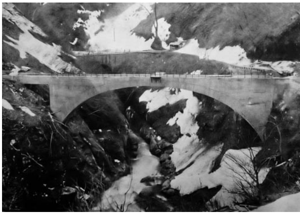
Megane Arch Bridge (Yonesaka Line, Yamagata Pref.) (Civil Engineering, 1935)
