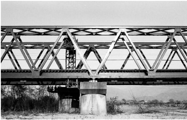
Intermediate support of the three-span continuous truss of Saigawa Bridge (Author)
