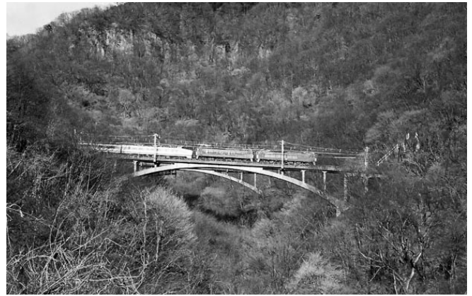
Abandoned Usuigawa Bridge with max. span of 70 m as RC railway arch bridge on 66.7‰ grade (Author)
