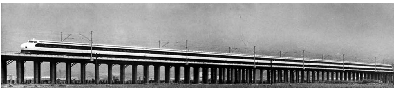
Tokaido Shinkansen viaduct, 1965 (The Railway Museum)
