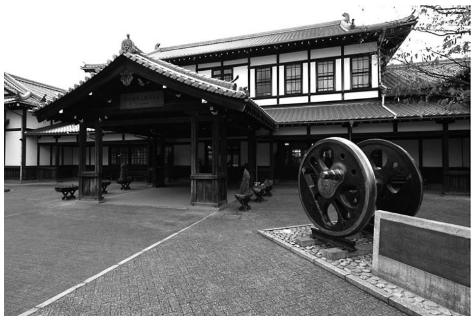
Umekoji Steam Locomotive Museum Exhibition Hall (former Niijo Station)
