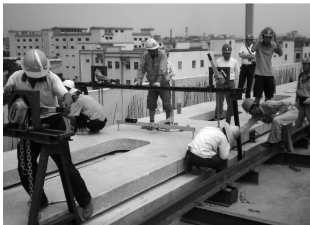
Laying (left) and completed (right) test slab track
