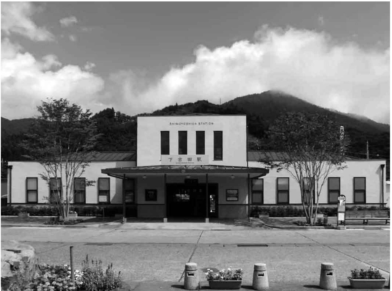
Front of renovated Shimoyoshida Station
