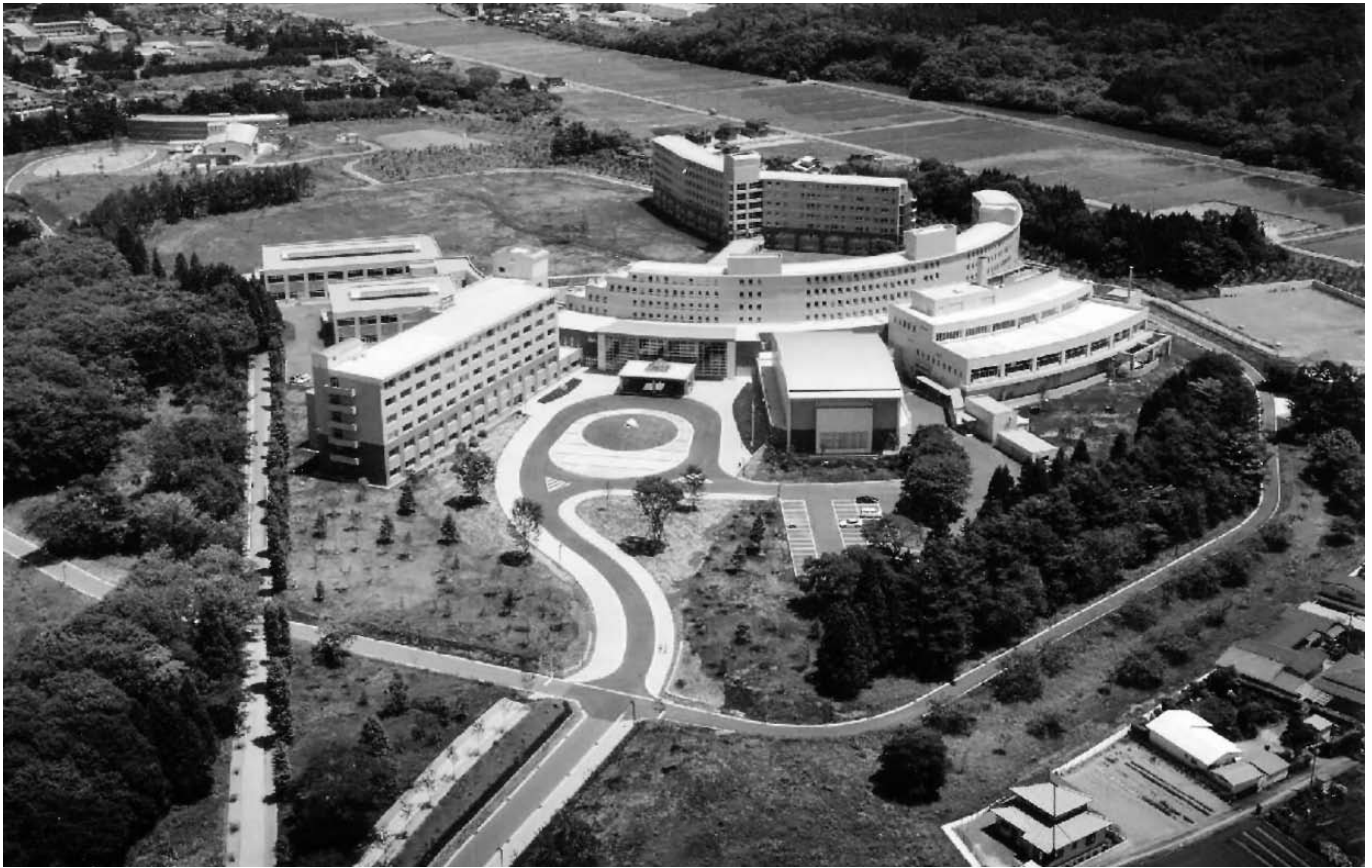
JR East General Education Center in Shirakawa City
