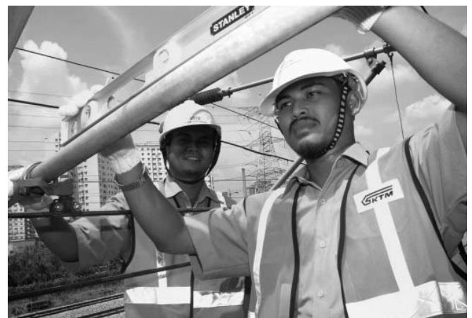
Maintenance of overhead catenary requires skilled employees (KTMB)
