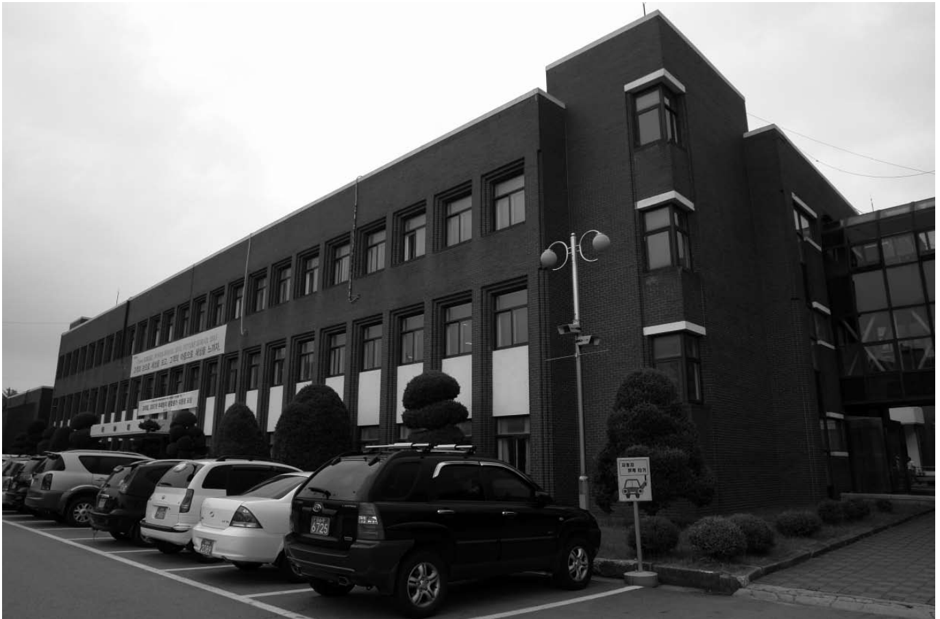
Auditorium and lecture building of International Railway Training Center
