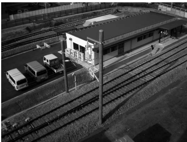
Part of practice line under construction
