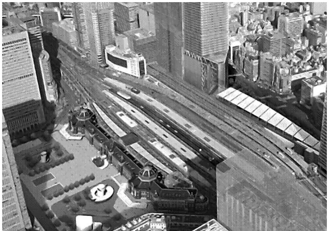
Solar panels to be installed on platform roofs as part of major renovation works of Tokyo Station
