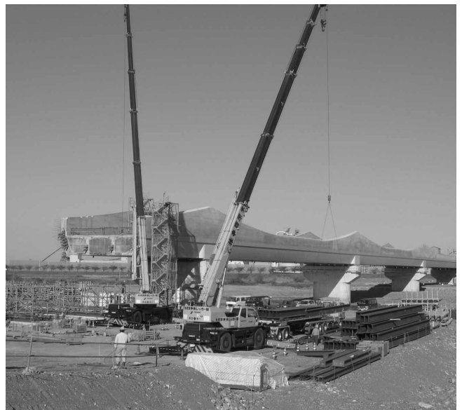
Construction of elegant 7-span Himekawa Bridge on Hokuriku Shinkansen
