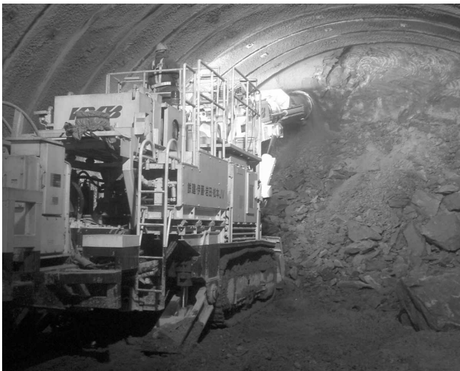
Boring Oshima-Tobetsu Tunnel on Hokkaido Shinkansen
