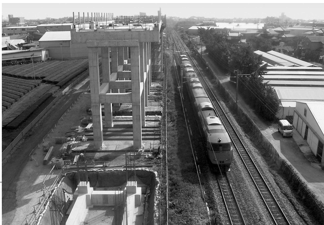
Relay Tsubame passing Chikugo Kumano Viaduct under construction on Kyushu Shinkansen
