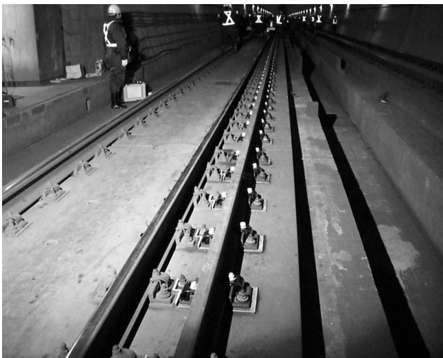
Dual-gauge tracks in Seikan Tunnel
