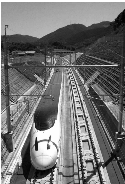
Kyushu Shinkansen running on ladder track
