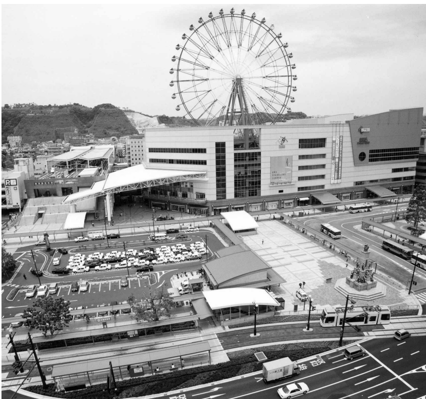
Development of station buildings and plaza at Kagoshima-Chuo Station for opening of Kyushu Shinkansen
