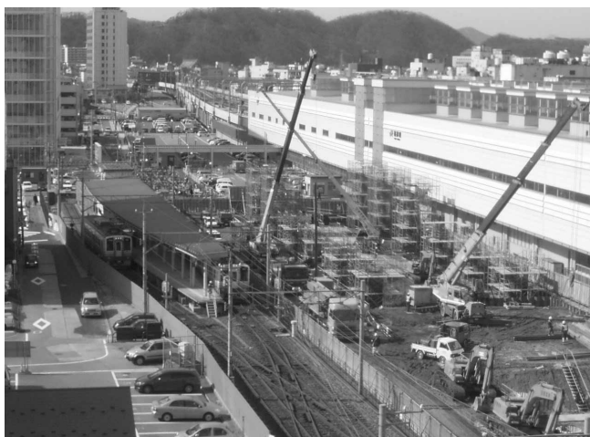
Station for new shinkansen line under construction
