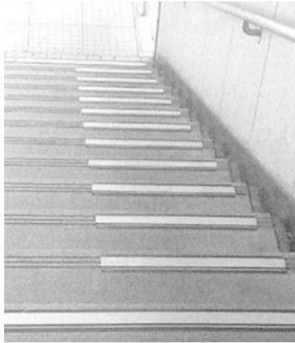
Staircase level-difference seal at Doro Station on Tohoku main line (JR East)
