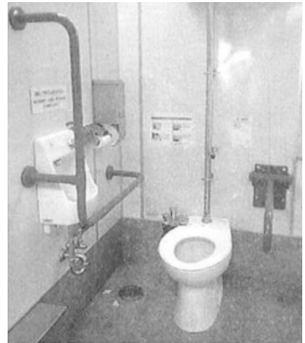
Interior of multifunction toilet at Nisshin Station on Kawagoe Line (JR East)
