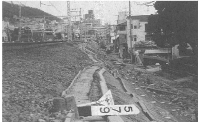
Ballasts being run out of track due to disruption of slope at Settsu Motoyama–Sumiyoshi section on Kobe Line. (JR West)
