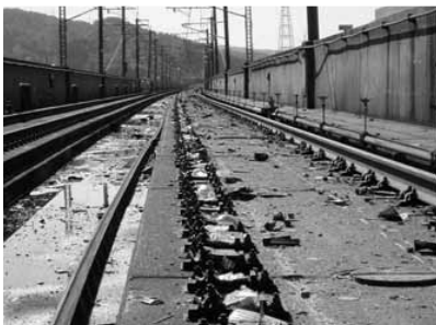
Damage to track caused by passage of derailed Toki 325
