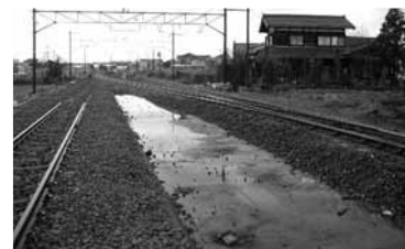
Installed turnout (Echigo Takiya Station)
