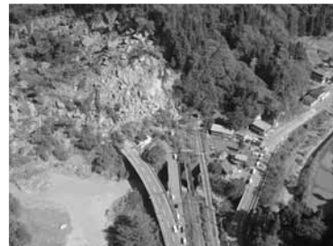
Landslide blocking Enoki Pass Tunnel portal
