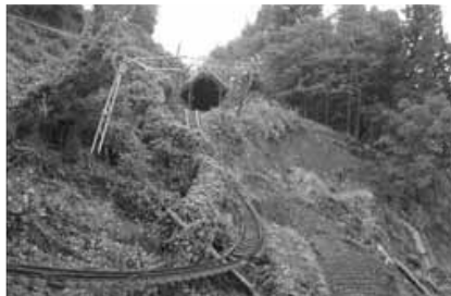
Collapsed embankment (220 km 500 m from base)
