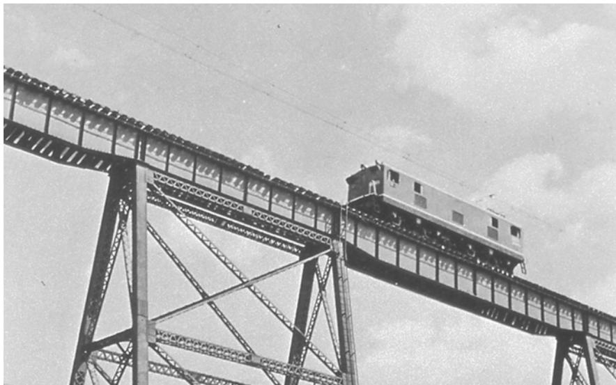
AC Electrification of Senzan Line using ED44 Electric Inspection Car
