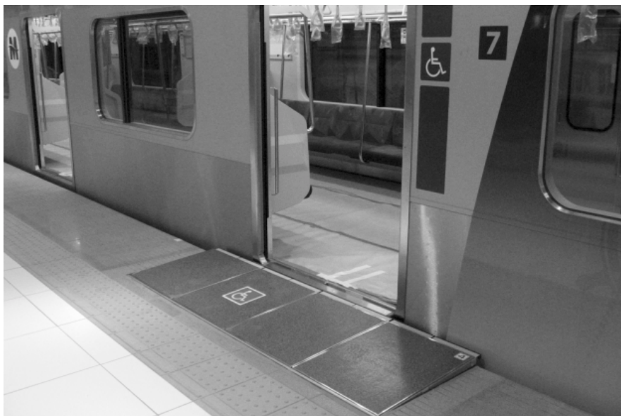
Ramp to eliminate gap and step for wheelchair users
