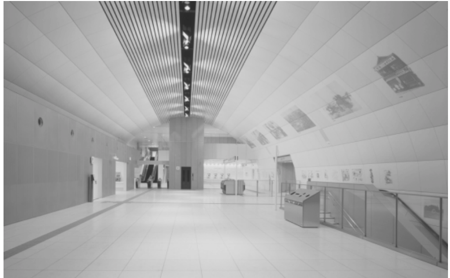
Concourse to first station platform on line at Motomachi-Chukagai Station
