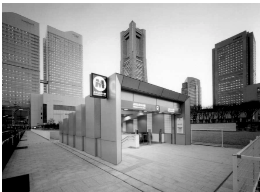
Tactile tiles provide guidance to stations
