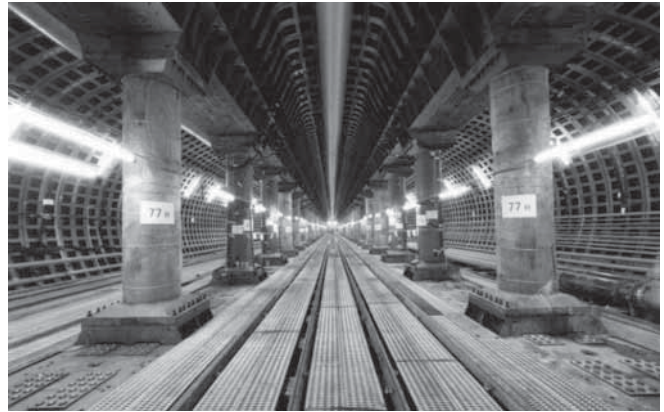
Station structure at Iidabashi Station (E06)
