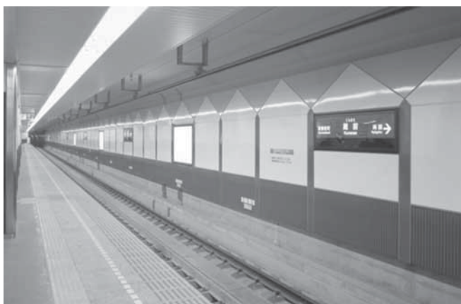
Trackside wall at Kuramae Station (E11)
