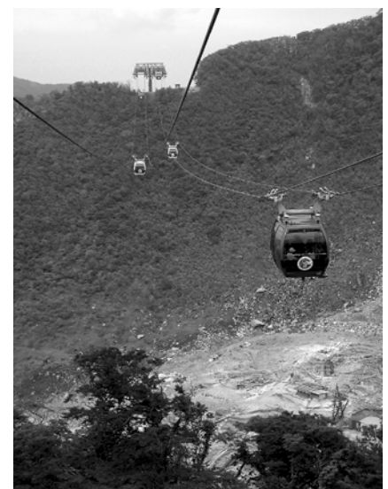
Harunasan Ropeway using two linked gondolas. This fixed mono-cable pulse ropeway in Gunma Prefecture features linked gondolas with a simple structure like a ski lift to cut costs. (Y. Kuroda)
