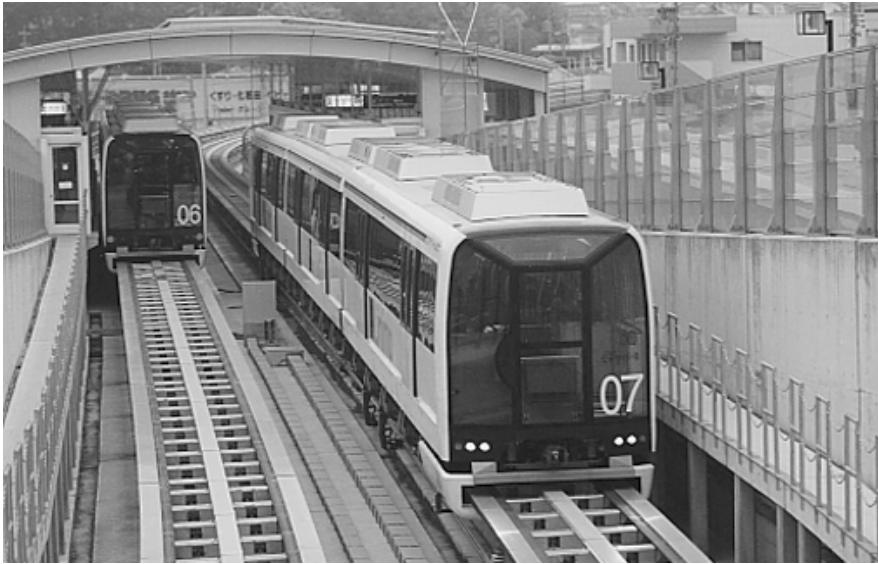
Aichi Rapid Transit's for Linimo levitating 6 mm above the track. This is Japan's first magnetic levitation system for commercial service, carrying more than 10 million people to the Aichi Exposition by July 2005. (Author)
