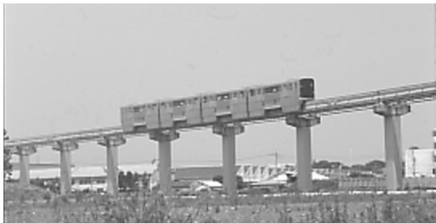
Tokyo Tama Intercity Monorail running between redevelopments in West Tokyo. This monorail on the western side of Tokyo acts as a link between three radial commuter lines running from Shinjuku. The track is built mainly over roads and developed land but there are some tunnels on sections through the Tama Hills. (Author)
