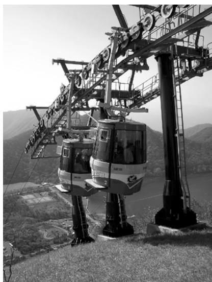
The Hakone Ropeway has recently been upgraded to become Japan's first Funitel system using a wider gondola and a double-loop mono cable, resulting in higher stability during windy conditions and a more comfortable ride. (Y. Kuroda)
