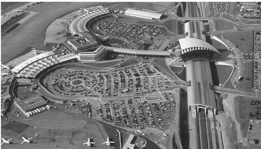
View of TGV station and terminals at LYS (SNCF)
