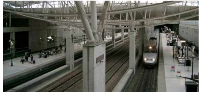
TGV Station in CDG (SNCF)
