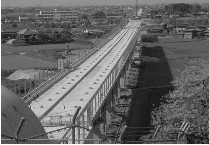
Takadatajiri Viaduct under construction (JR TT)
