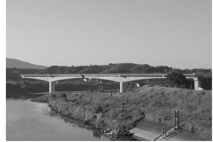
Kikuchi River Bridge under construction (JR TT)
