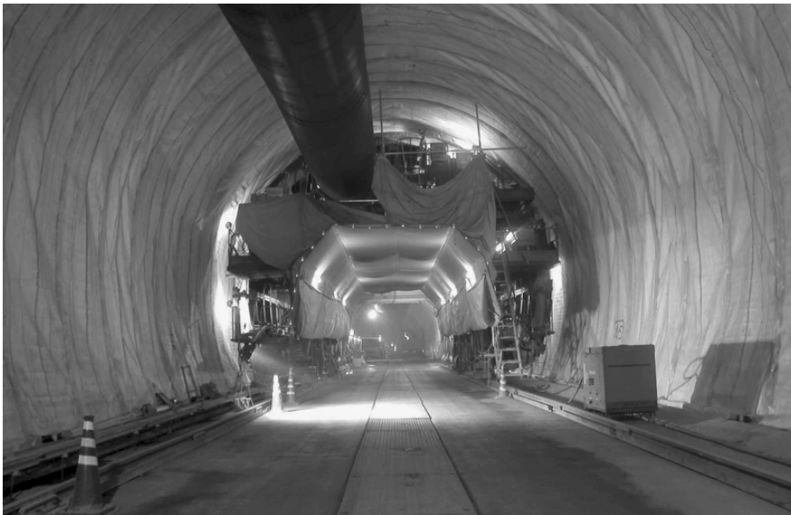
Iiyama Tunnel (22.2 km) nearing completion
