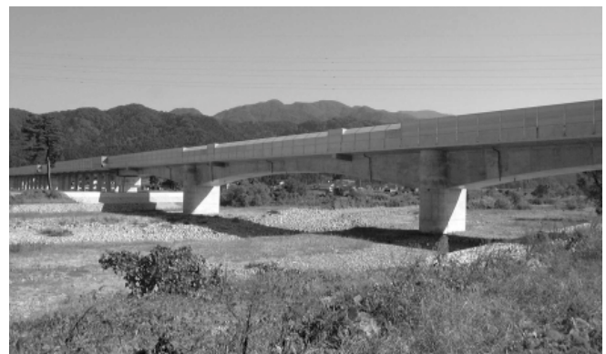
Ogawa River Bridge (JRJT)
