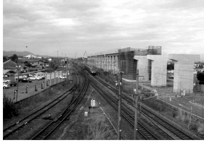
Uto Viaduct under construction (JR TT)
