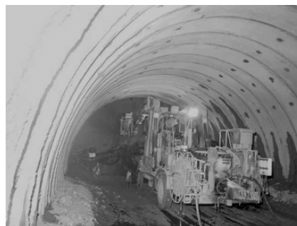
Hakkoda Tunnel (26.5 km) under construction (JRJT)
