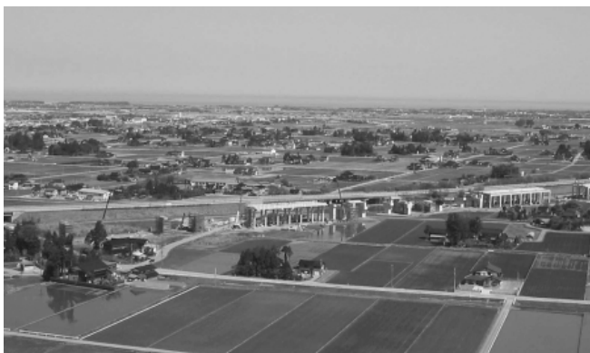
Viaduct under construction for Shin Kurobe Station (provisional name) (JRJT)
