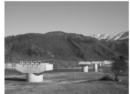
Supports for No. 5 Chikuma River Bridge (JRJT)
