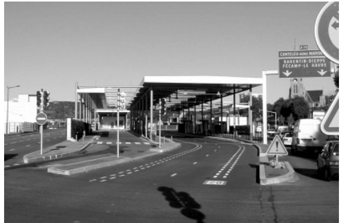
Segregated right of way at Mont Ribouidet on lines T1, T2 and T3 of Rouen TEOR (TCAR)
